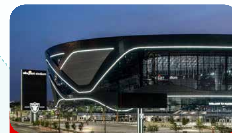
Allegiant Stadium NEVADA, USA
